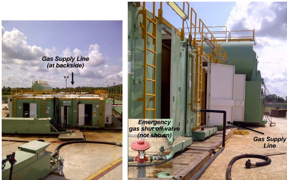
**Figure 4 Generator House, Gas Supply Lines, and Shut-Off Valve**
