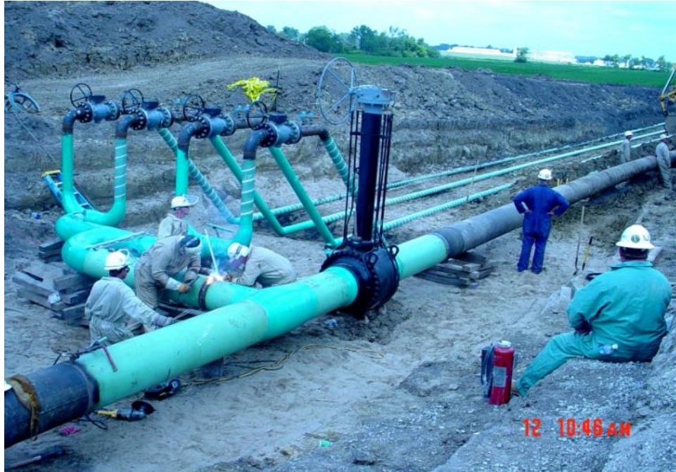
Figure 3 Direct Injection Scavenger System under Construction
