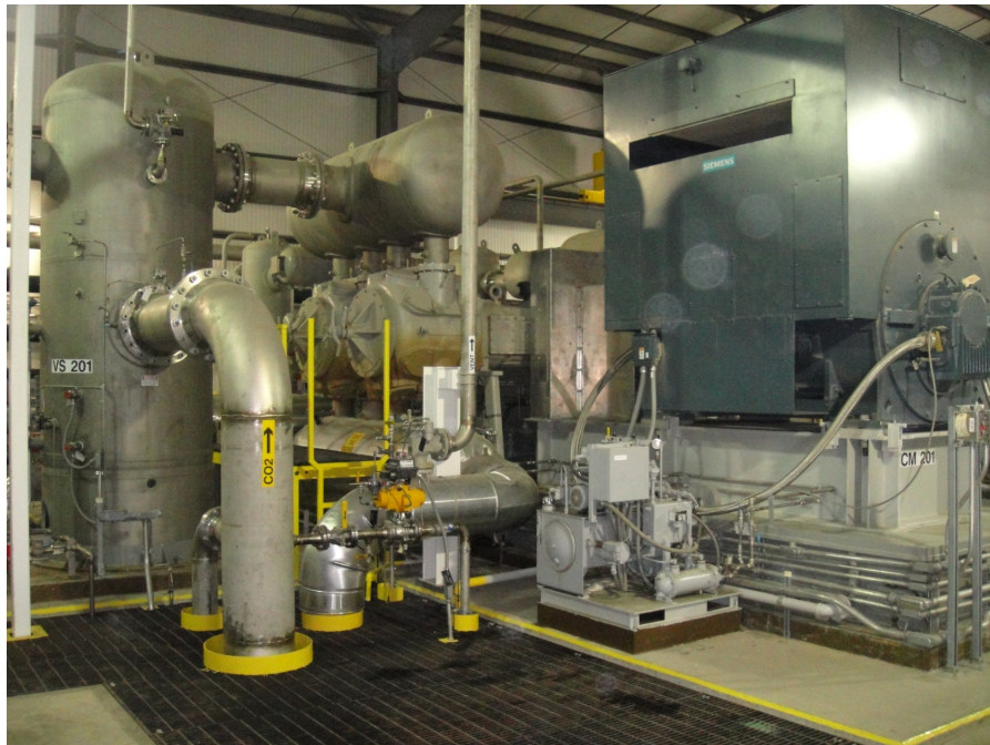
Figure 4 – Reciprocating Compressor
