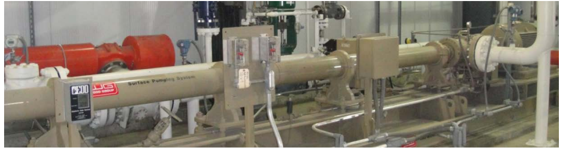
26-Stage, 200 hp (149 kW) Centrifugal Pump
