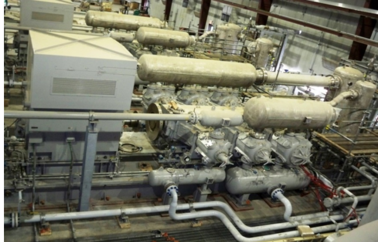
Chaparral Coffeyville 50 MMscfd / 1 MM tonne/yr 19,500 hp (14.5 MW) CO 2 Compression and Dehydration Facility
