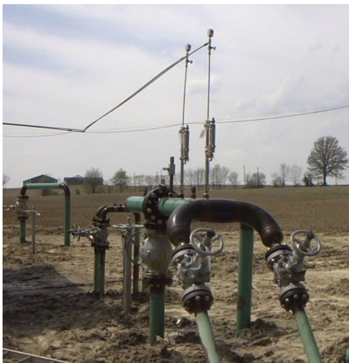
Figure 18. 3 in. Double Pipe DI Unit in southern Illinois
