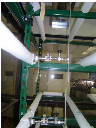
Figure 10. Sampling Port Connection
