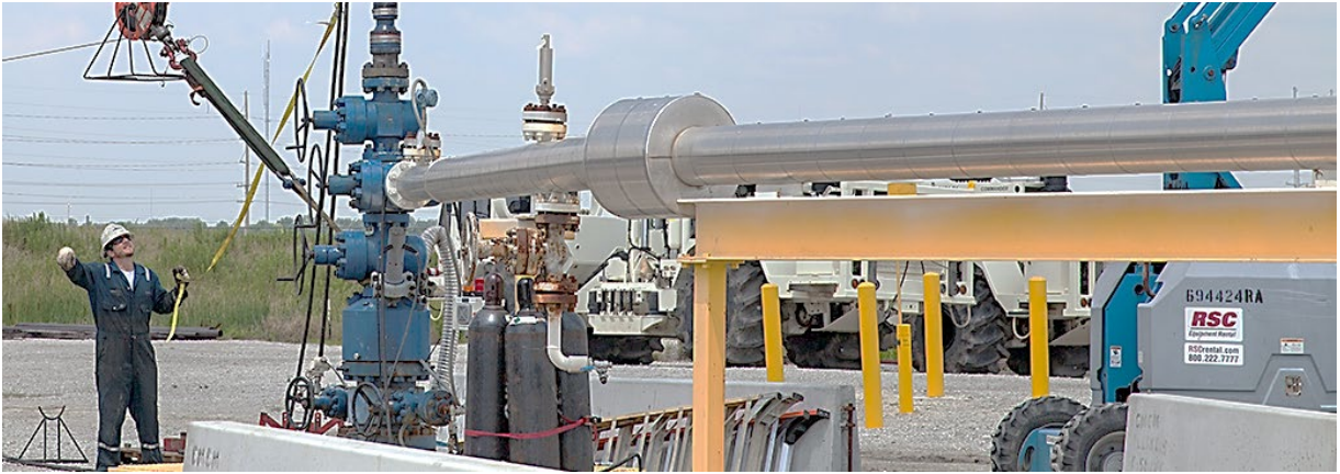
Fig. 3. Illinois Basin-Decatur Project Above-Ground, Insulated Injection Pipeline, 150 mm diameter, 2 km, Schedule 40 API 5L X52 Carbon Steel.
