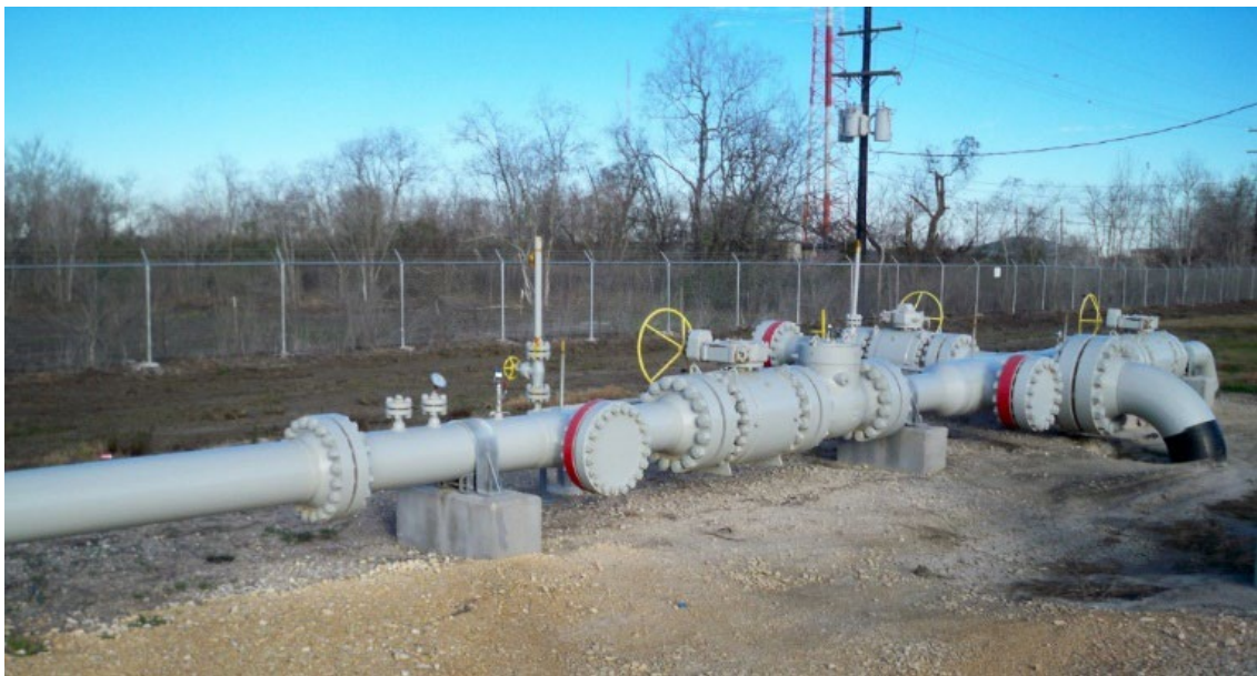
Fig. 2. 400 mm diameter commercial CO 2 pipeline at above / below ground transition.
