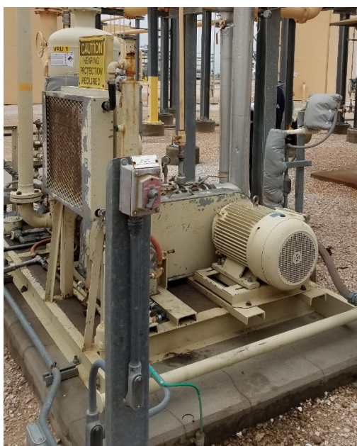
Figure 7. Example VRU Screw Compressor.
