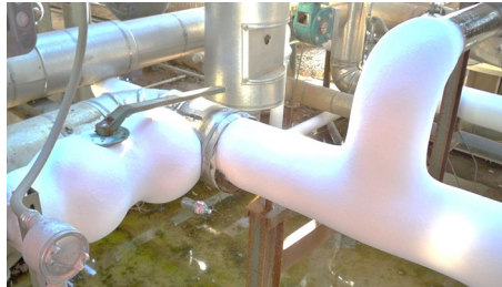
Water Vapor from the Air Freezes on Pipe Before Insulation is Installed.
